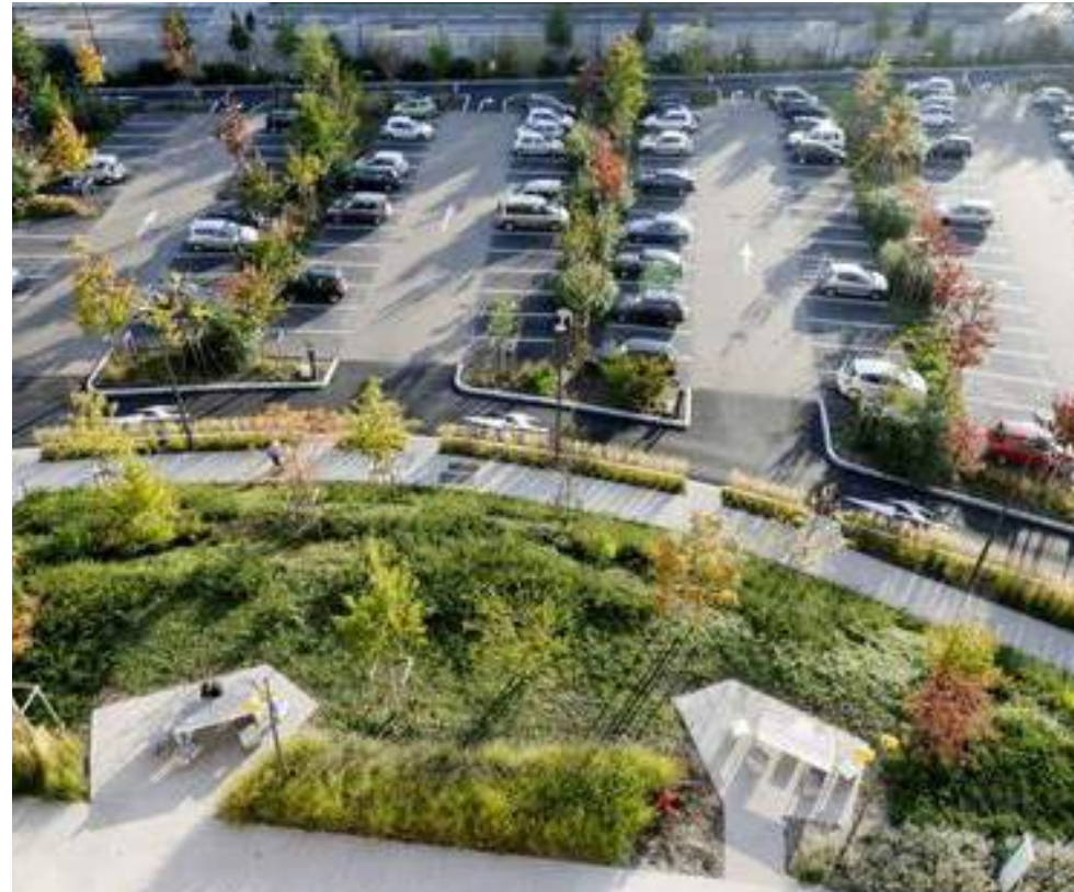
Create a sense of arrival. Hospital Hautepierre | France Even in the parking lot, visitors should know they are in a park.
